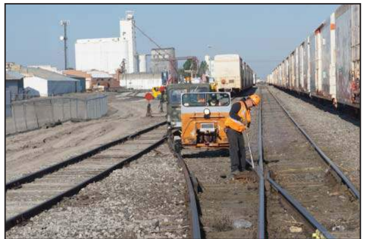
Making the transition to the main line, motorcar operator Bill Evens waits for Sean Crowe to adjust the troublesome spring frog.
