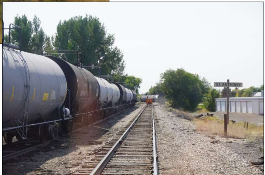
St Anthony station -oil cars on side tracks.
