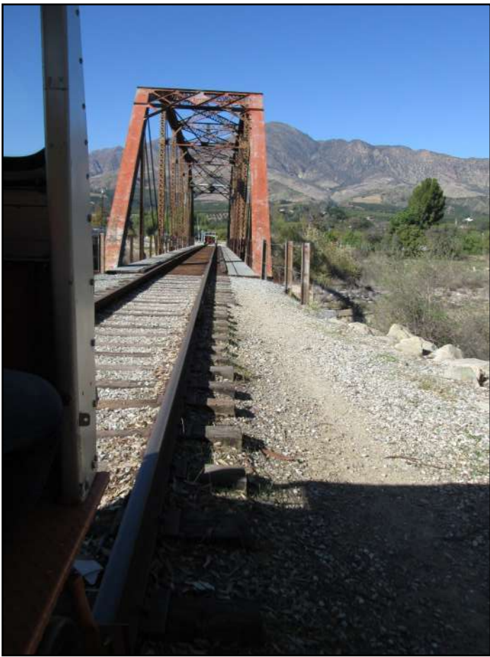
Sespe Creek Bridge built in 1902.
