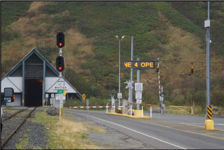
As we wait on the Whittier side, the tunnel light tells us when the tunnel is next open in this direction.
