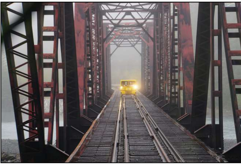
Bridge at Snow River MP 14.5.
