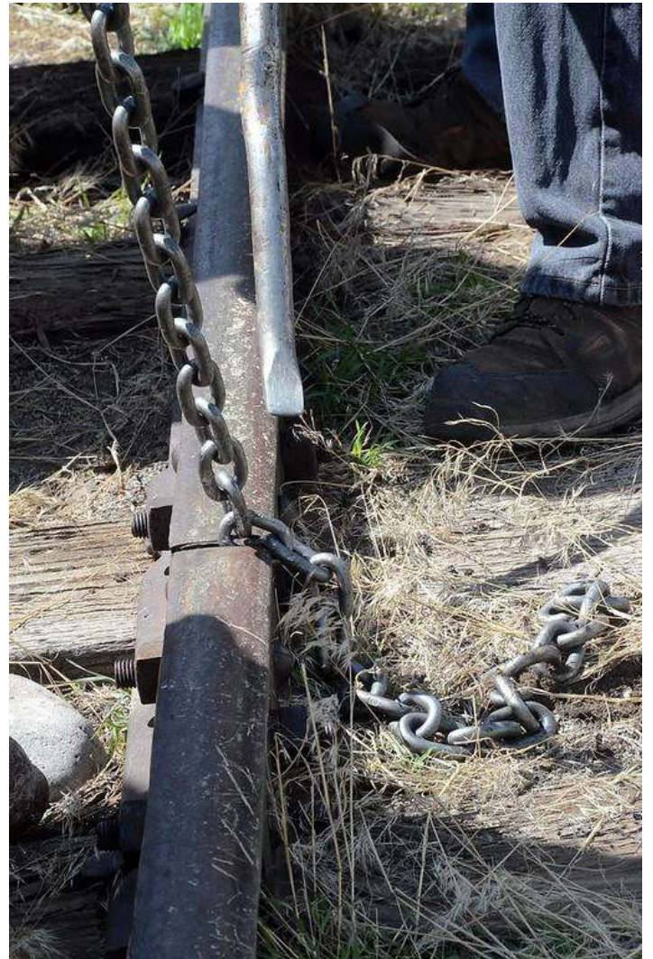
Working to free a chain brake after the track expanded in the warm sun.
