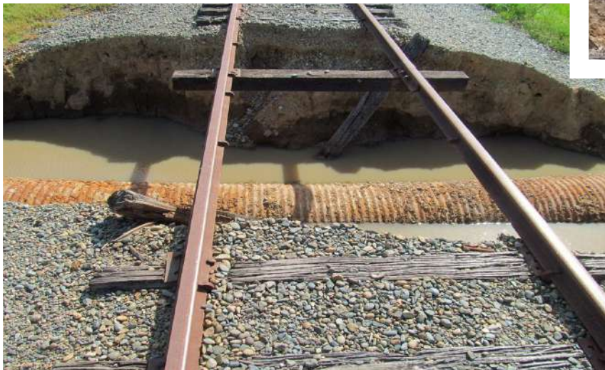
Slow down thar! A very slow and careful crossing allowed everyone to make it safely across the washed out section of track. The track was repaired soon after with the help of MOW volunteers.
