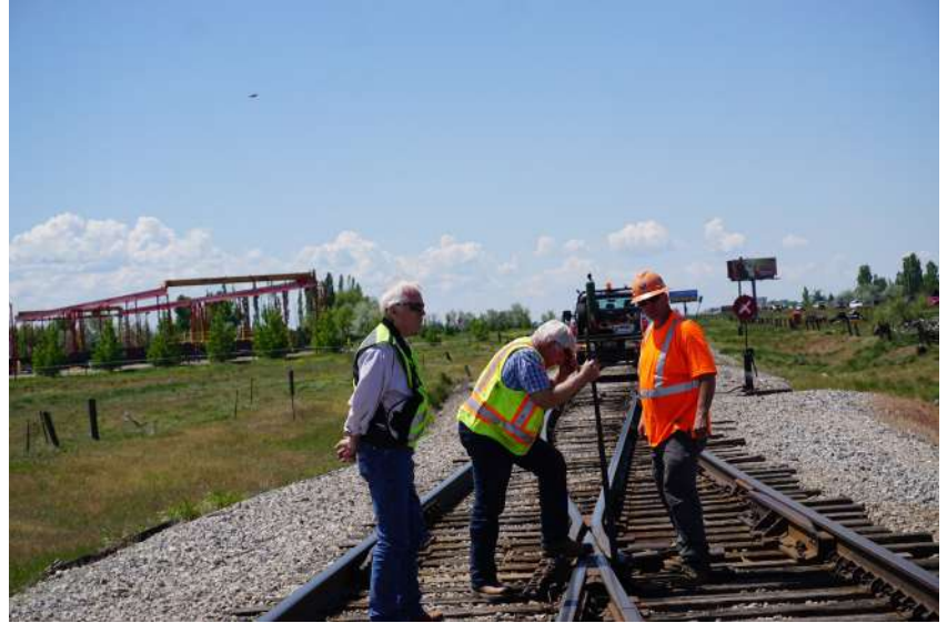
Propping open the spring frog: Dave Balestreri & railroad escort with guest on-looker.
