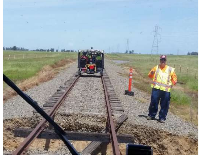
Slow down thar! A very slow and careful crossing allowed everyone to make it safely across the washed out section of track. The track was repaired soon after with the help of MOW volunteers.
