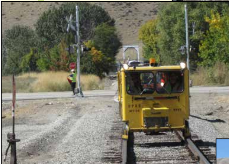
Crossing the Payette River and Highway 55, the MOW group entered the Horseshoe Bend Rail yard.
