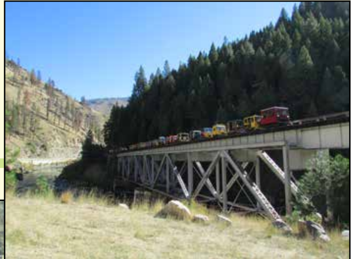
Half way between Banks and Big Eddy, the MOW group posed their motorcars on the Payette River open deck truss bridge.
