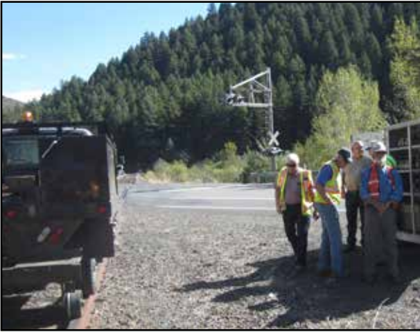
Friends of the Joseph Branch crew wait at Minam to activate the Highway 82 crossing signals.
