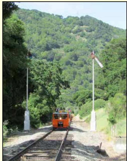
The excursion splits the semaphore signal in the depth of Niles Canyon.
