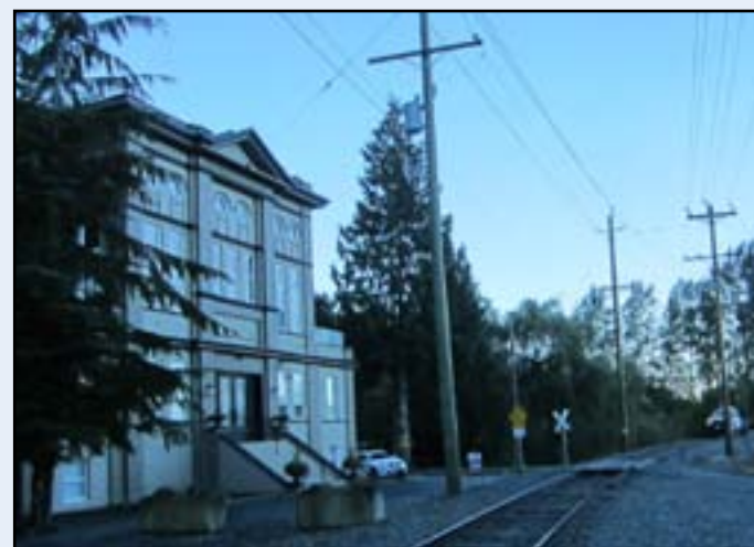
The excursion, lead by the Southern Railway of British Columbia hi-rail truck approach the Sumas Substation.
