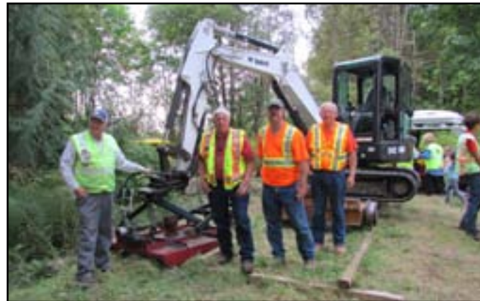
John Martin, Dave Balestreri, Don Wigen and Ken Creasy inspected the brush cutting equipment used by the Fyfe Volunteer Section Gang that groomed 30 miles of right of way for the excursion.
