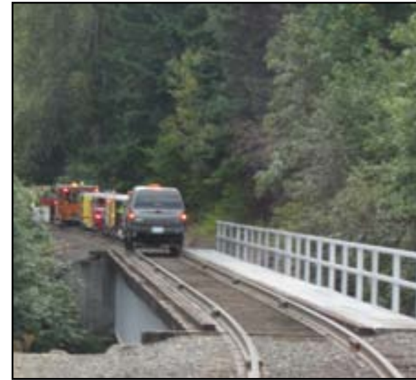
Crossing over the East Fork of the Hood River.
