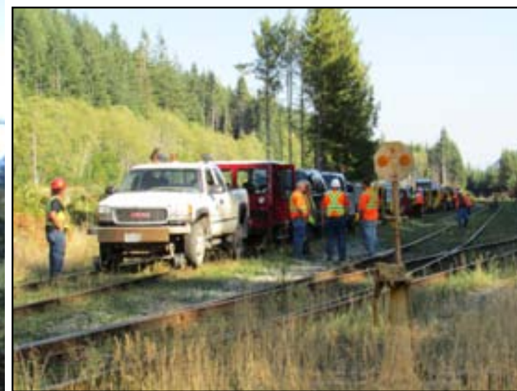
The final afternoon comfort stop was held at Siding 4 milepost 29. This is a log-reloading area used by log-carrying helicopters for transferring its log loads to rail cars. Timber stands to be harvested on the surrounding steep mountainsides are inaccessible by road. Helicopters are employed to lift the logs from the logging site and transport them to Siding 4. The two siding tracks can hold up to 100 log cars.
