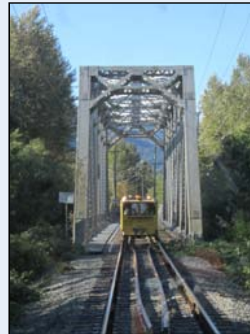
Southern Railway of British Columbia Vedder River Crossing.
