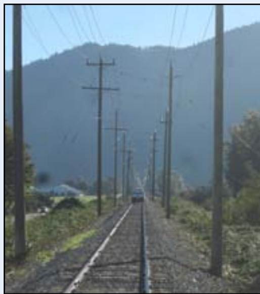
Ahead of the excursion group is Vedder Mountain. The poles gracing the right of way are the remnants of what was the British Columbia Electric Railway's trolley wire.
