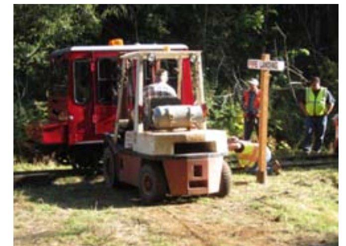
Ken Fyfe positioned the repaired motorcar back on the rails.
