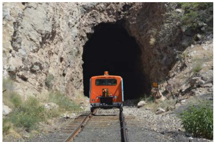
The excursion enters the west portal of the Middle Butte tunnel.
