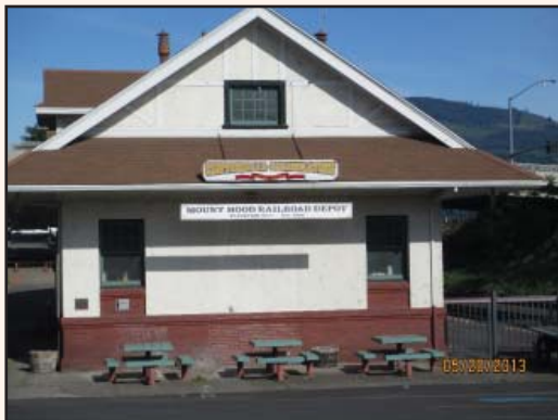
A local group purchased the Union Pacific branchline in 1987 with the rail line again being sold in 2008 to Permian Basin Railways. The ex Union Pacific depot is now used as the Mount Hood Railroad headquarters.
