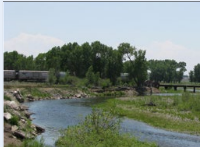
The Rio Grande River crossing.
