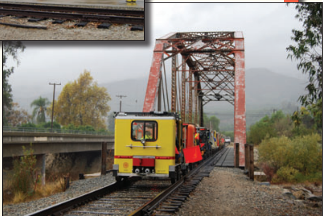
A photo stop at the 1901 Sespe Creek Bridge.
