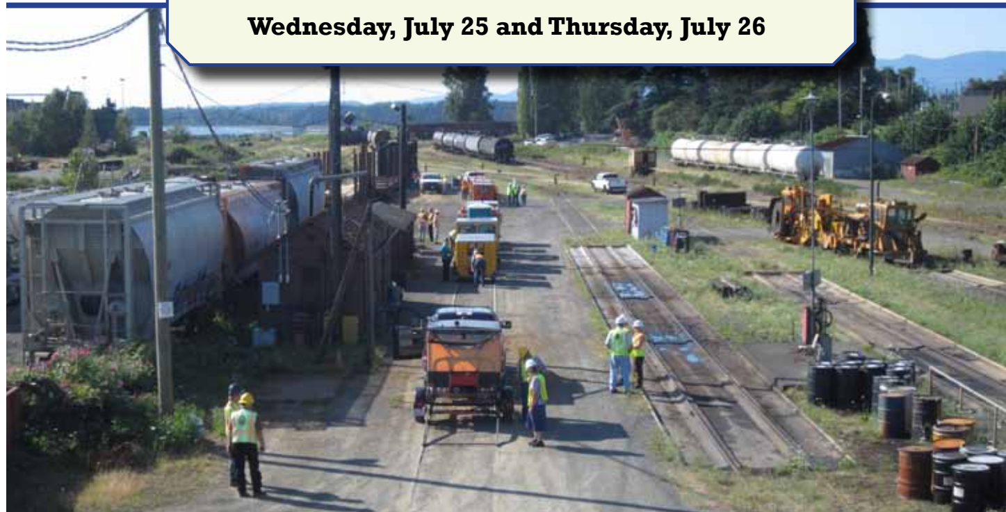
The Southern Railway of Vancouver Island's Wellcox yard is located on Nanaimo's waterfront and served as the motorcar set on site. This view was taken from the Case Street bridge shows Dave Balesteri and Don Wigen in the lower left hand corner supervising the set on activities.
