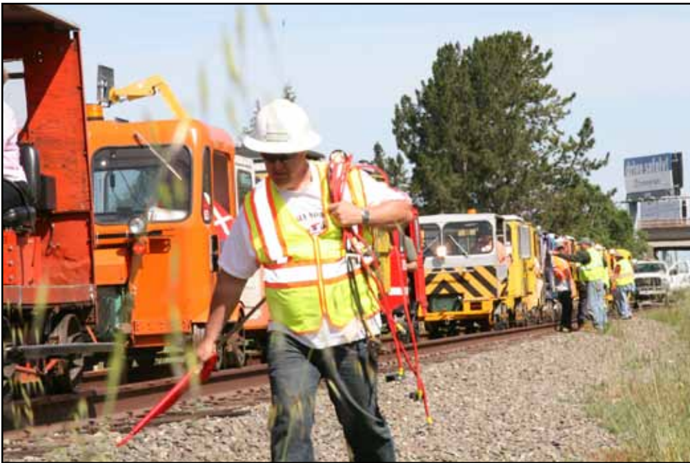
Pete Mihelcic of Summit Signal busy picking up highway crossing shunts and carrying them forward to be used at southbound crossings. He and his brother Danny volunteered to help protect the excursion through more than 50 highway crossings between Healdsburg and Petaluma.
