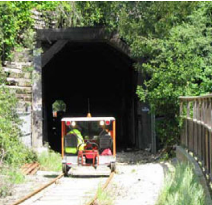
Motorcars enter the Mission Hill Tunnel located in downtown Santa Cruz. The 972 feet long bore was excavated in 1880.
