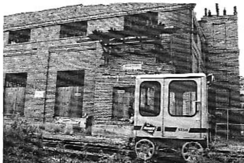
TOP: Bill Evans and Bud Knedler pose near Denton, MT. Bud is one of the directors of the Central Montana Railroad. Bottom: This substation once supplied power to the wire on the Milwaukee Road's main line near Royal City, WA. Ron Zammit's Tomah Cab MT-19 poses in front. Ron Zammit
